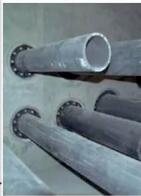
Cable trench in transformer room Service-runs within sub-structure of building
