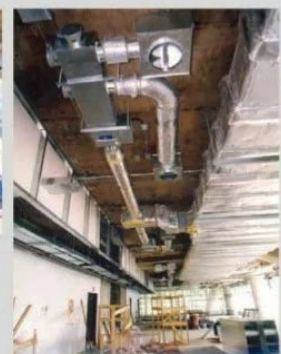
Ceiling services before the laying of false ceiling
