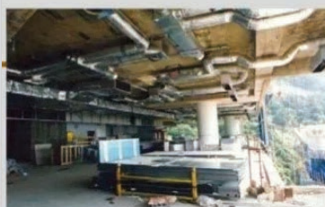
Ceiling services before the laying of false ceiling
