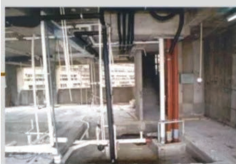
Provision of opening and pipe-run for bathroom in residential building
