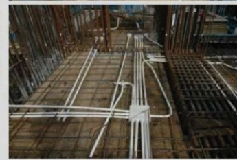
Service-runs inside floor slab
