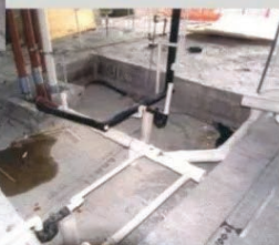
Ceiling services before the laying of false ceiling
