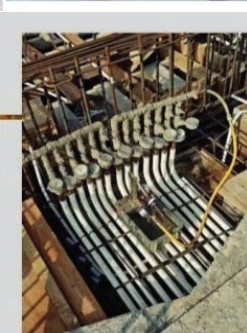
Service-runs inside floor slab
